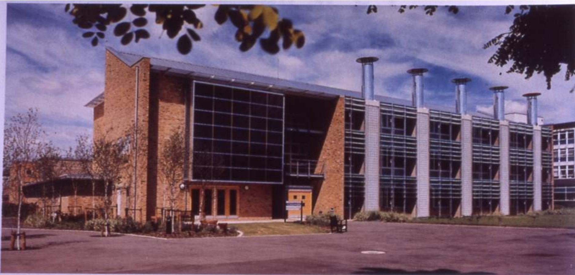
Figure 1. The south facade of the BRE Environmental Building. External motorized fritted glass louvres can be adjusted to screen out solar gain, or, on overcast days, admit sky luminance. The louvres are controlled automatically to follow the sun's movement.
