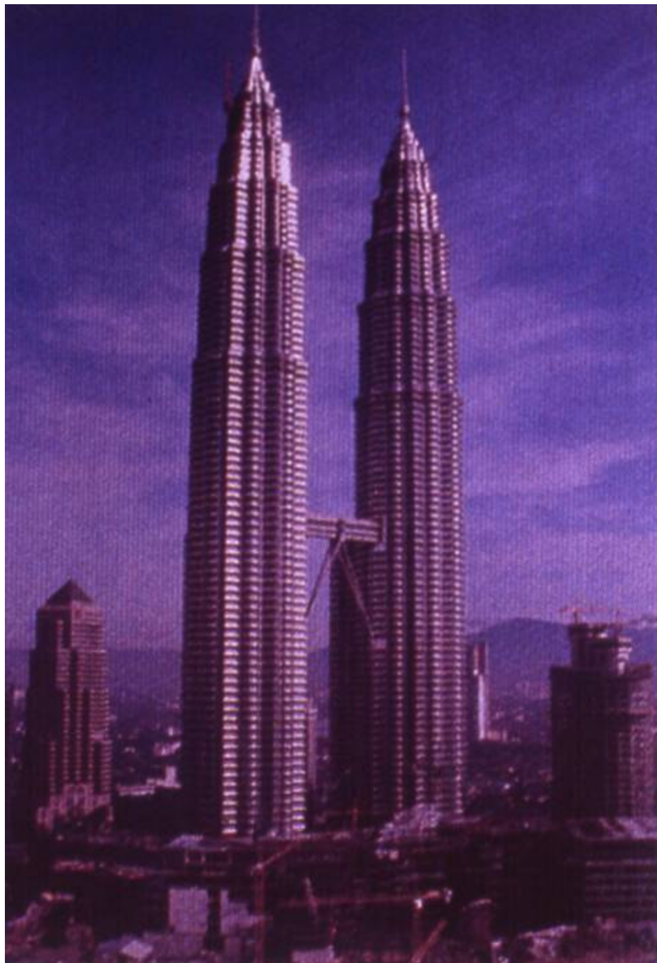
C. Pelli, Petronas Towers Kuala Lumpur, Malasia, 1997
