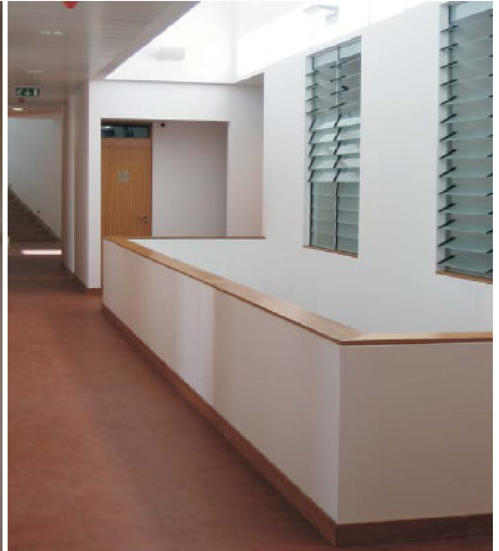
Adjustable glazed venetian blinds for ventilation
