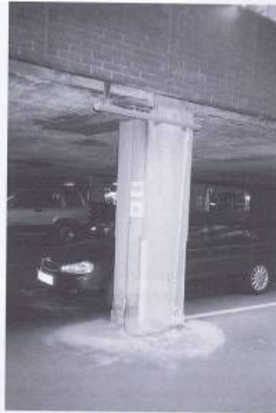
Fig. 4.6(a) Poor maintenance of this car park has led to the formation of a stagnant water where the inadequate drainage keeps water off cars but does not cure or control leakage from the floor above.
