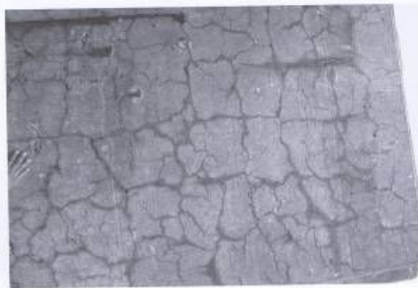
Fig. 4.5 Map cracking due to an alkali-silica reaction.
