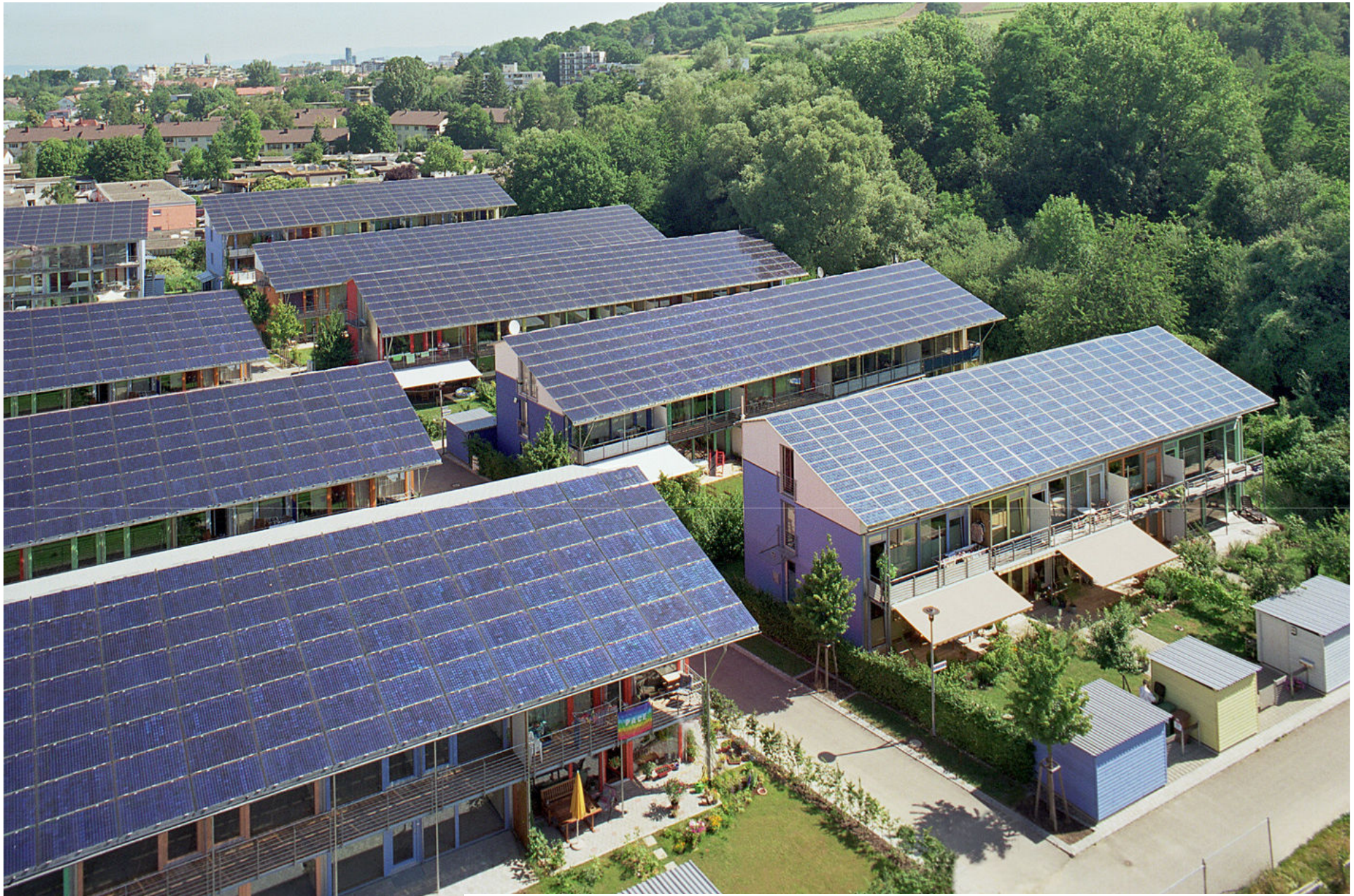
Solar Settlement Freiburg, Germany Architecture and Concept: Rolf Disch
