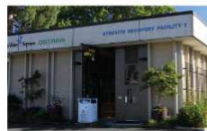
Clean Water Services' Nutrient Recovery Facility at the Tigard Advanced Wastewater Treatment Plant in Tigard, Oregon
