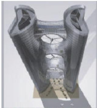
View Tower 3 side view with three turbines (M&P), University of Stuttgart
