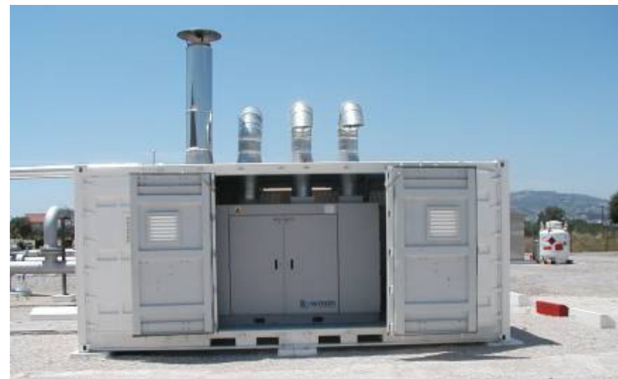
Microturbina Bowman de 80kWe (400V)
