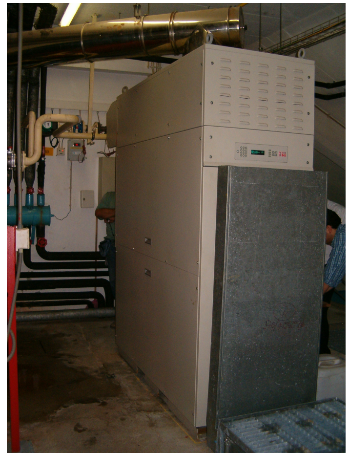
Microturbina Capstone de 60kWe (400V)
