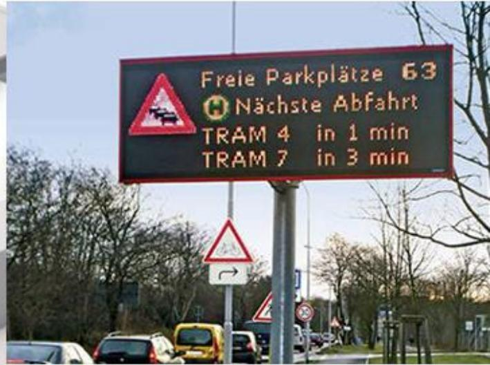
In Halle, Germany, more than 50 percent of drivers have switched to trams since the introduction of an intermodal traffic concept. The system informs drivers of the current traffic situation and free parking spaces as well as the departure time of the next tram. As a result, the intelligent networking of Sitraffic system modules has optimized traffic flow in the city of Halle and made using public transportation even more attractive.
